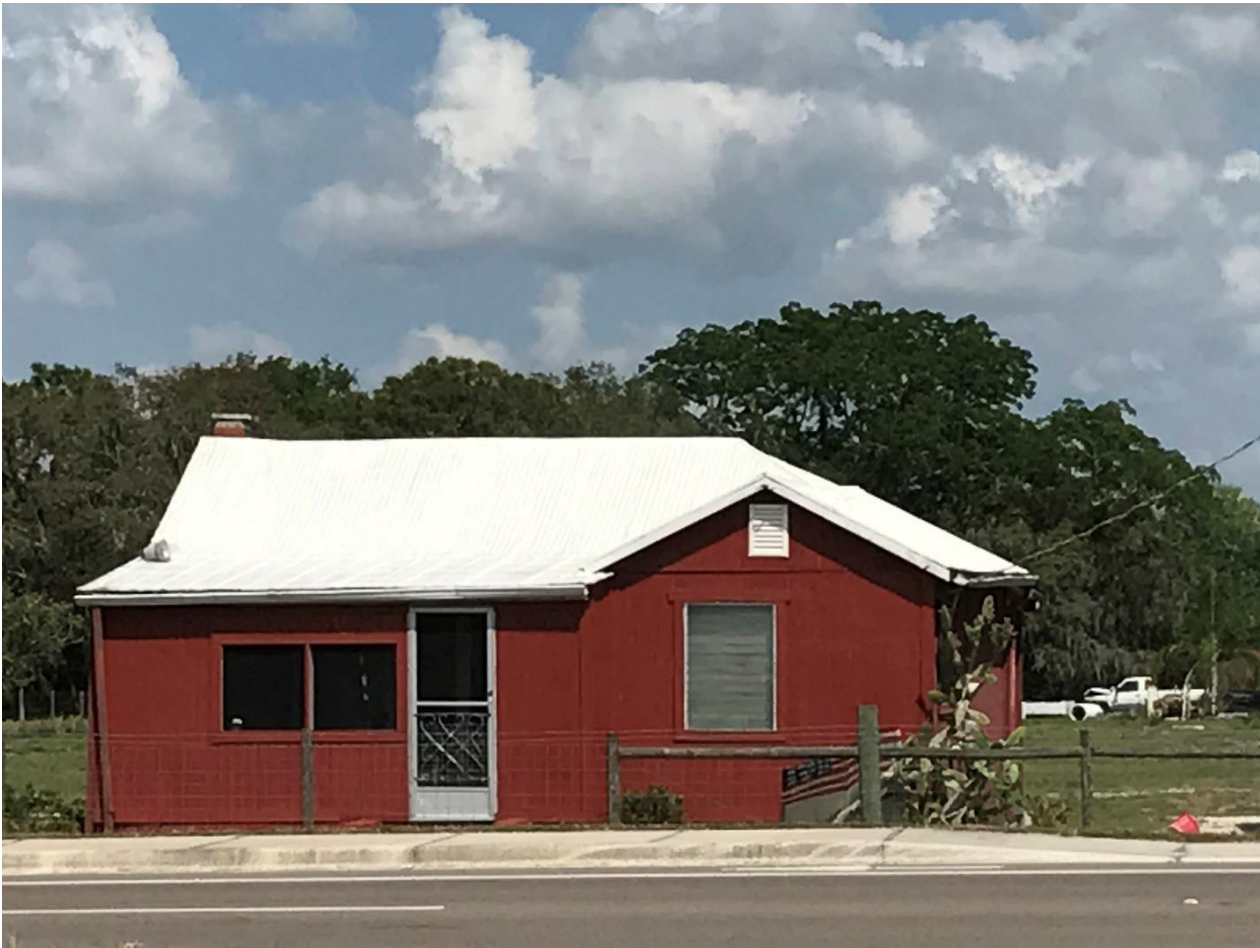
Example A: 879 square foot home, county assessed value at $39,134
